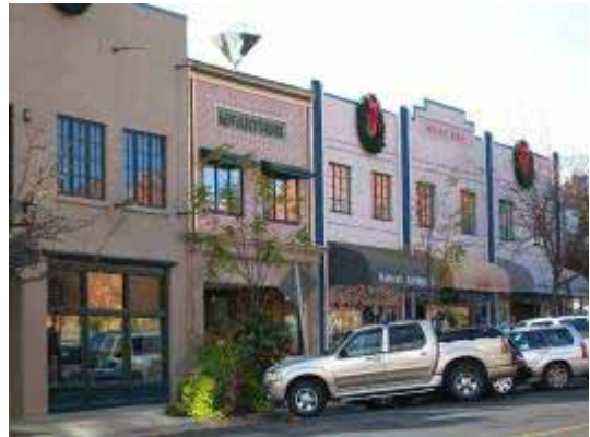
Example of two-part commercial block buildings with street level fenestration and details.
