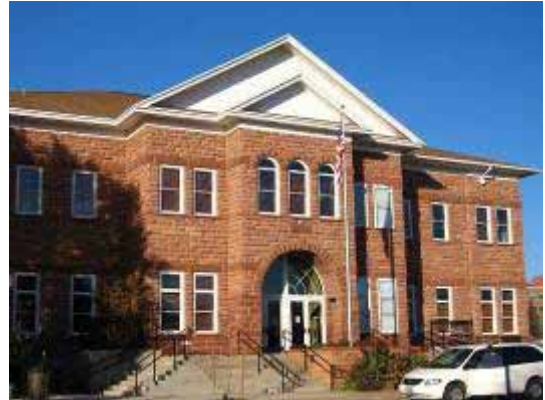
Example of central block with wings building form used for modern public library (2006).
