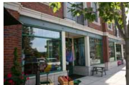
Fenestration of the façade at the ground level is the most important building element contributing to the quality of the pedestrian environment.
